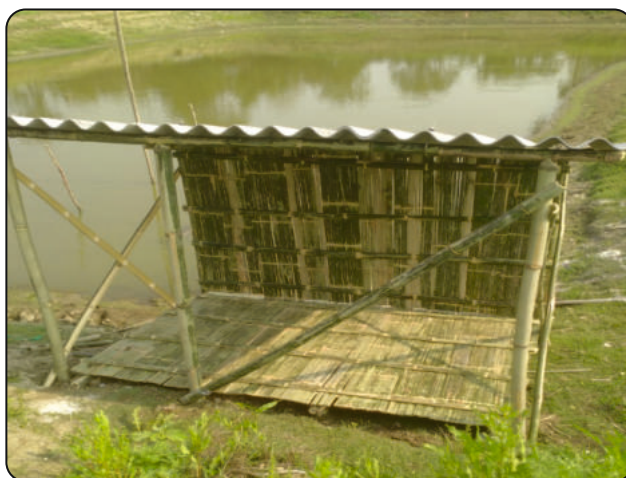
Fig. 8.17 Low-cost poultry house construction at Chandandighi
