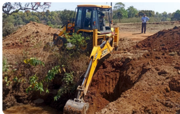
Fig. 8.9. Hapa ( Small pond) under construction
