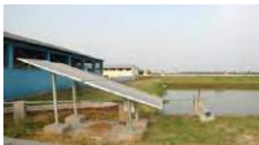
Fig. 4.8. Solar watering system for animal sheds
