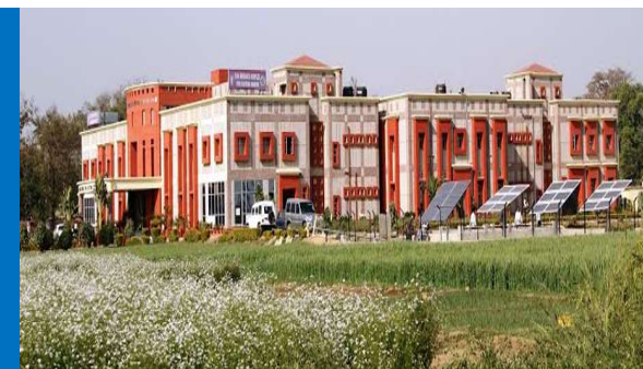
Administrative building cum Laboratory, ICAR RCER
